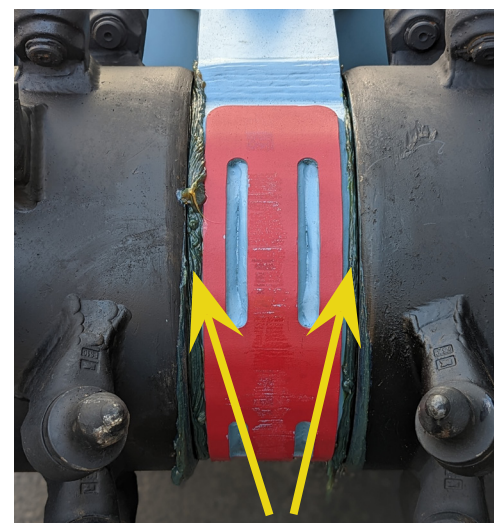
Proper greasing: coming out between the drum and housing
