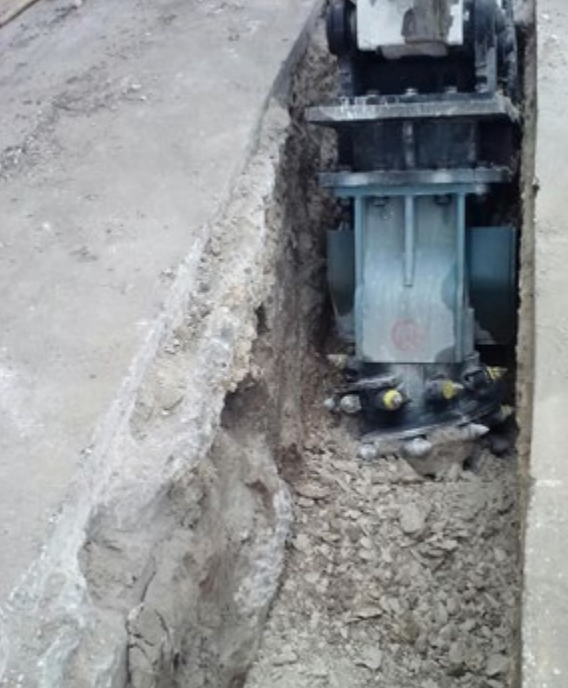
TC20 Digging a Utility Trench
